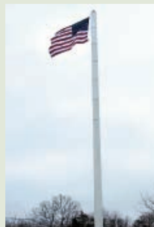
The Village Flag Pole serves as a revenue-producing cell tower.
